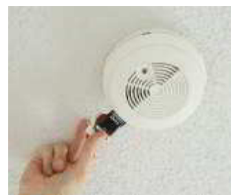
A smoke detector sounds an alarm when smoke enters its ionization chamber.
